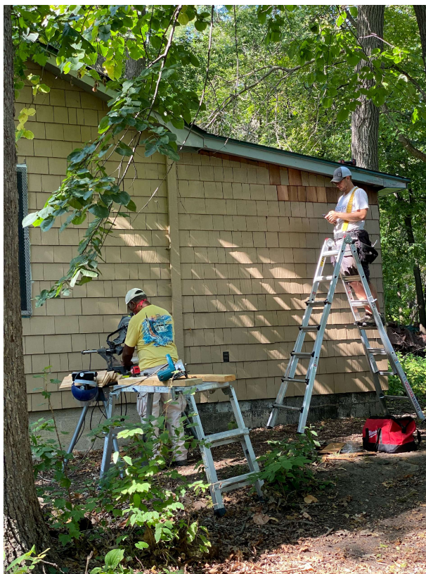
Jerry and Josh repairing Woodpecker damage to the Chapter House.
