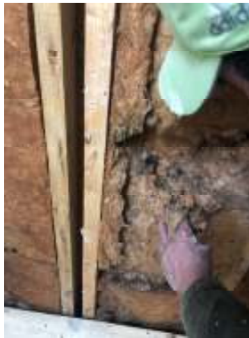
Removal of wet insulation, including a mouse nest and replacement of vapor barrier
